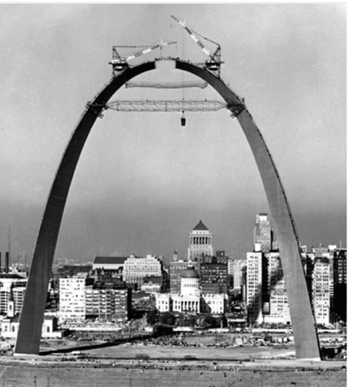
The Gateway Arch in 1965 nearing completion with custom-made lifts.
